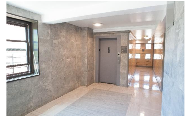
Renovated building entrance at Ocean Bay (Bayside)
