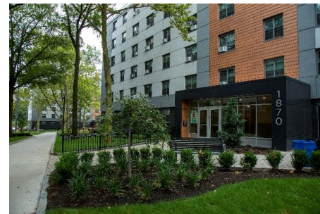
Site improvements at Baychester
