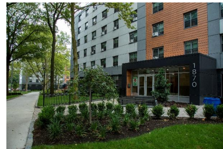
Site improvements at Baychester
