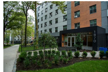
Site improvements at Baychester
