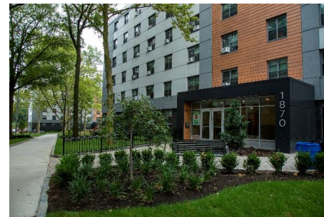
Site improvements at Baychester
