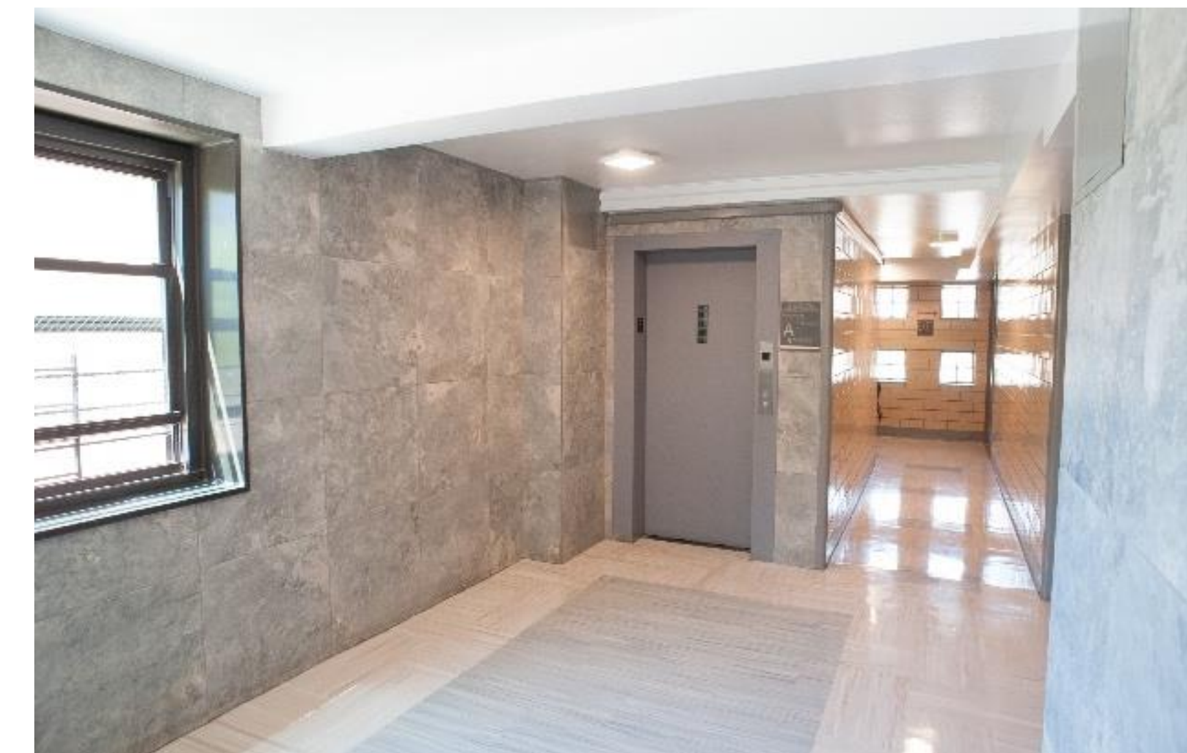
Renovated building entrance at Ocean Bay (Bayside)
