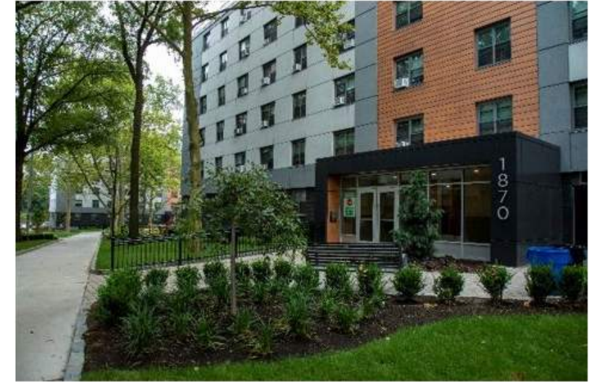
Site improvements at Baychester
