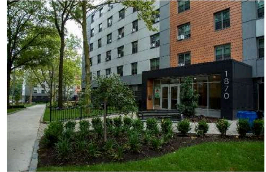
Site improvements at Baychester
