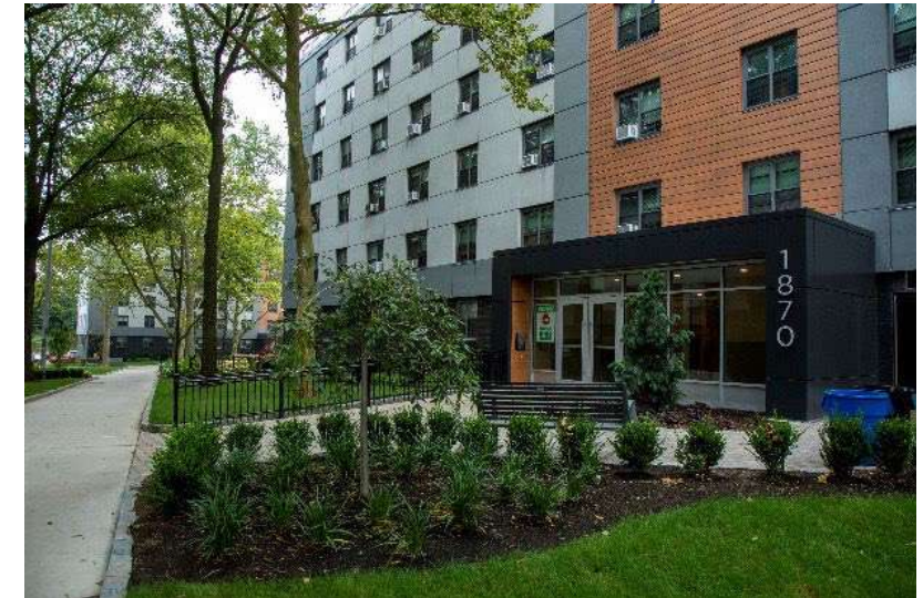
Site improvements at Baychester
