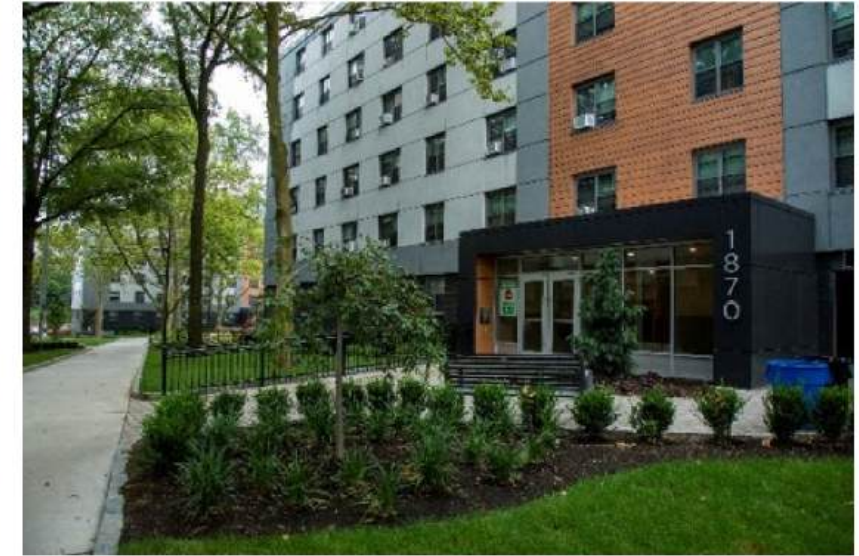
Site improvements at Baychester
