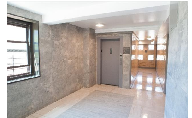
Renovated building entrance at Ocean Bay (Bayside)
