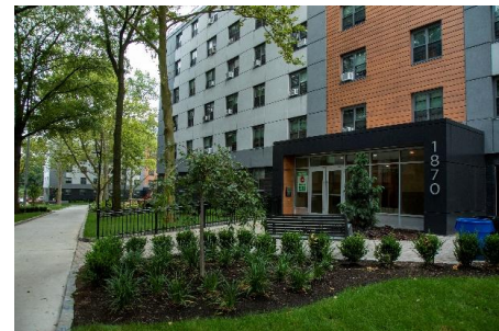
Site improvements at Baychester
