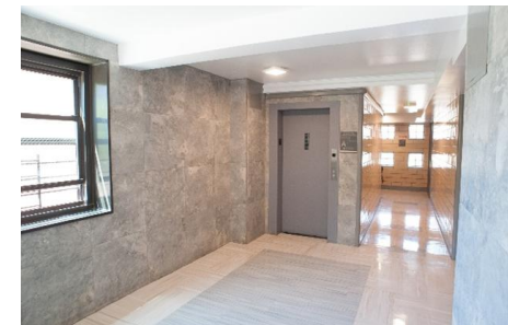
Renovated building entrance at Ocean Bay (Bayside)
